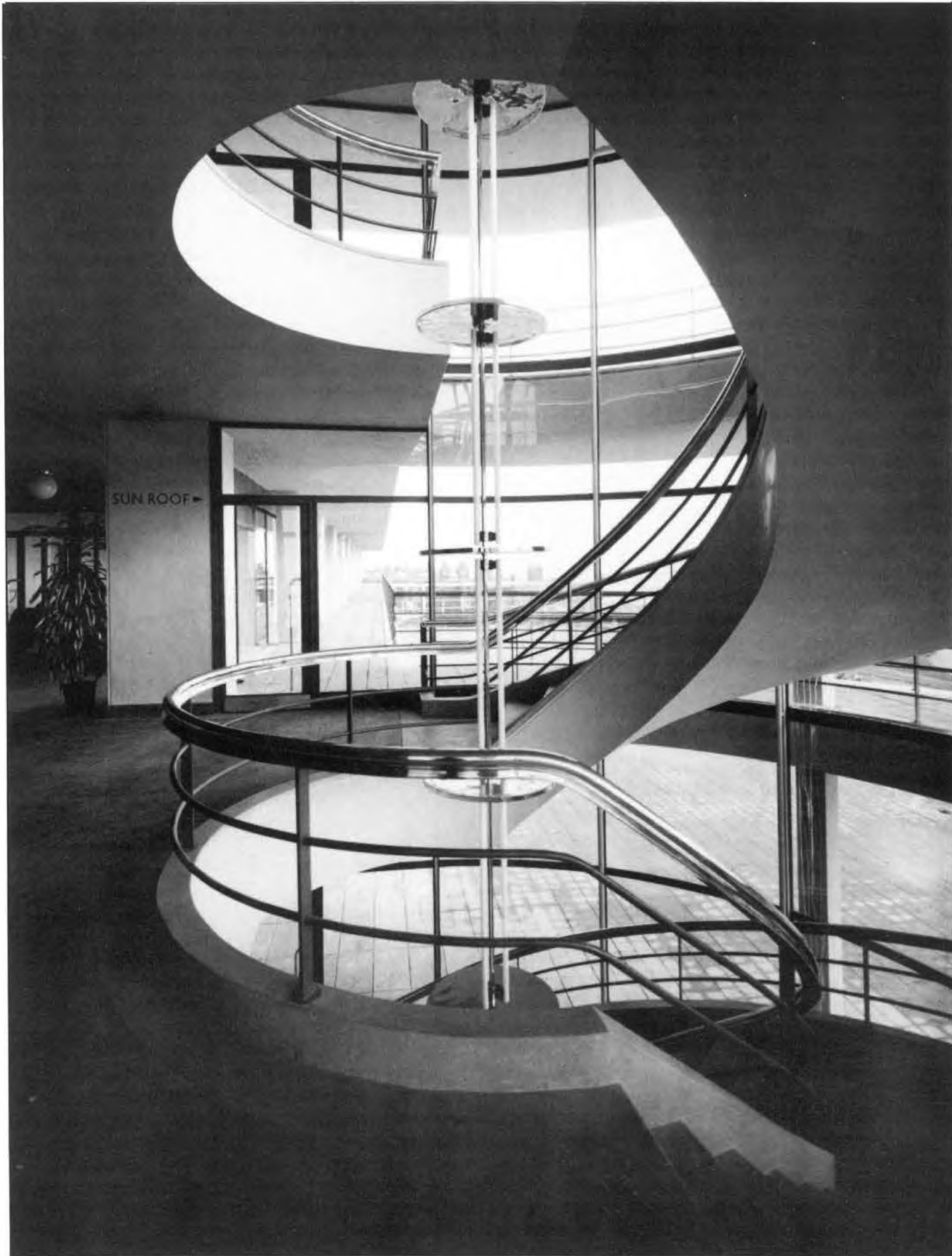
Staircase in the De La Warr Pavilion, Bexhill in 1937. [RCHM England]
